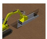
3) PERFORM DESIRED WORK, THEN PULL SHIELD FORWARD AND UP AT APPROPRIATE ANGLE AND REPEAT PREVIOUS STEPS AS NECESSARY.
