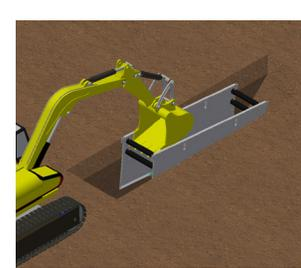
3) PERFORM DESIRED WORK, THEN PULL SHIELD FORWARD AND UP AT APPROPRIATE ANGLE AND REPEAT PREVIOUS STEPS AS NECESSARY.
